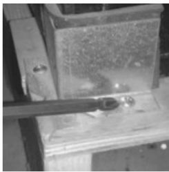
Image 1 Removing bracket from skid
